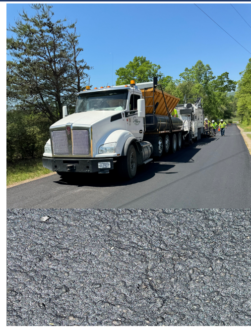
Pictured above: Applying surface course. Inset picture: Surface course texture.
