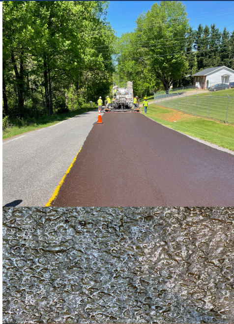
Pictured above: Applying scratch course. Inset picture: Scratch course texture.
